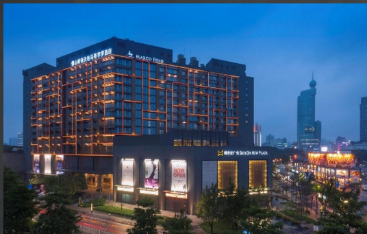
FOSHAN MAGOMEDRO HOTEL LOCATION: FOSHAN CHANCHENG SCALE: 30,000 SQUARE METERS DATE: 2016 CATEGORY: HOTEL
